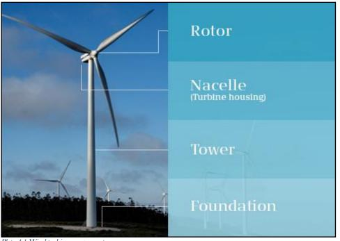
Plate 4-1 Wind turbine components
