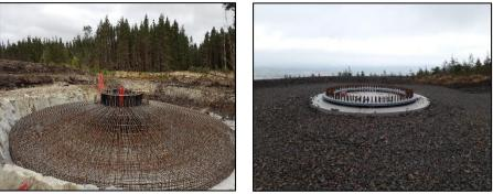
Plate 4-2 Turbine Base 'Anchor Cage'
