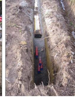
Plate 4-9 Typical Cable Trench View
