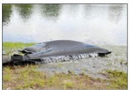
Plate 4-7 Silt bag under inspection
