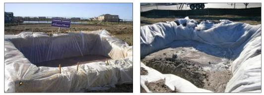
Plate 4-4 Concrete Washout Area
